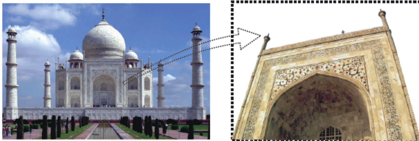
Figure 16.17: Taj Mahal and its corroded door
