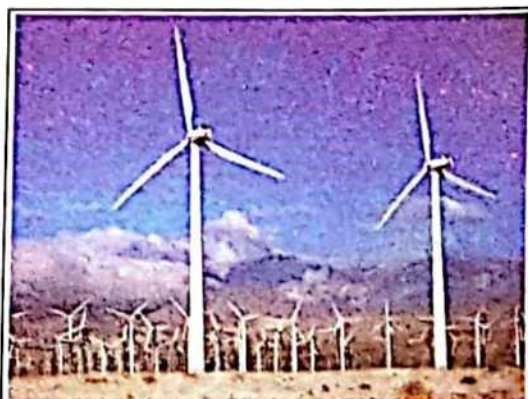
Wind Energy Farm: The Gansu wind farm in China is the biggest wind farm in the world. It generates up 7900 MW There are 7000 wind turbines in Gobi Desert.
