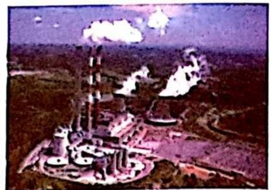
Fig.4.22: Coal thermal power plant
