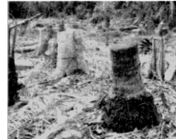
Figure: Chopping up of trees for the construction of road
